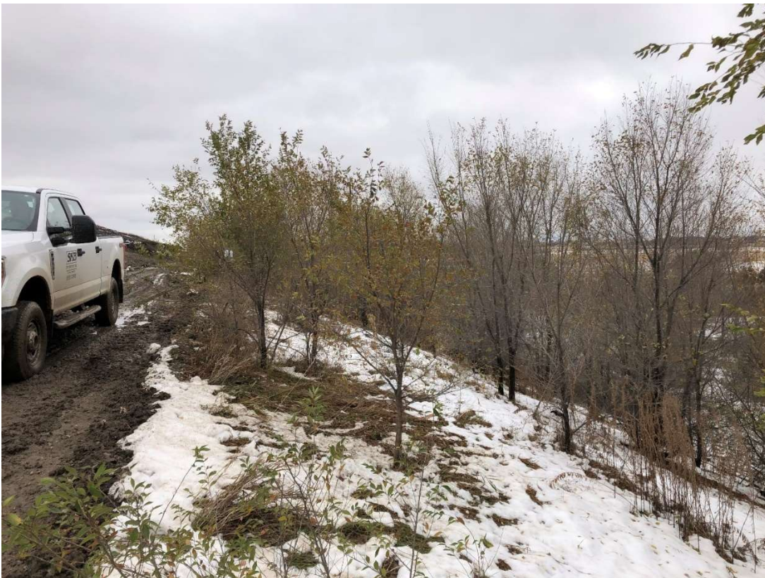
Location 8 – Looking Southwest, Cell 2C Southwestern Berm
