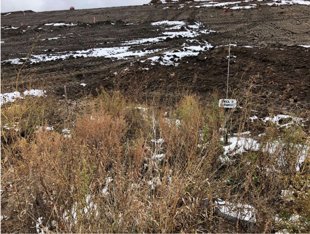
Location 6 – Looking Northeast, Southeastern Slope, Anchor Trench & New Liner Construction
