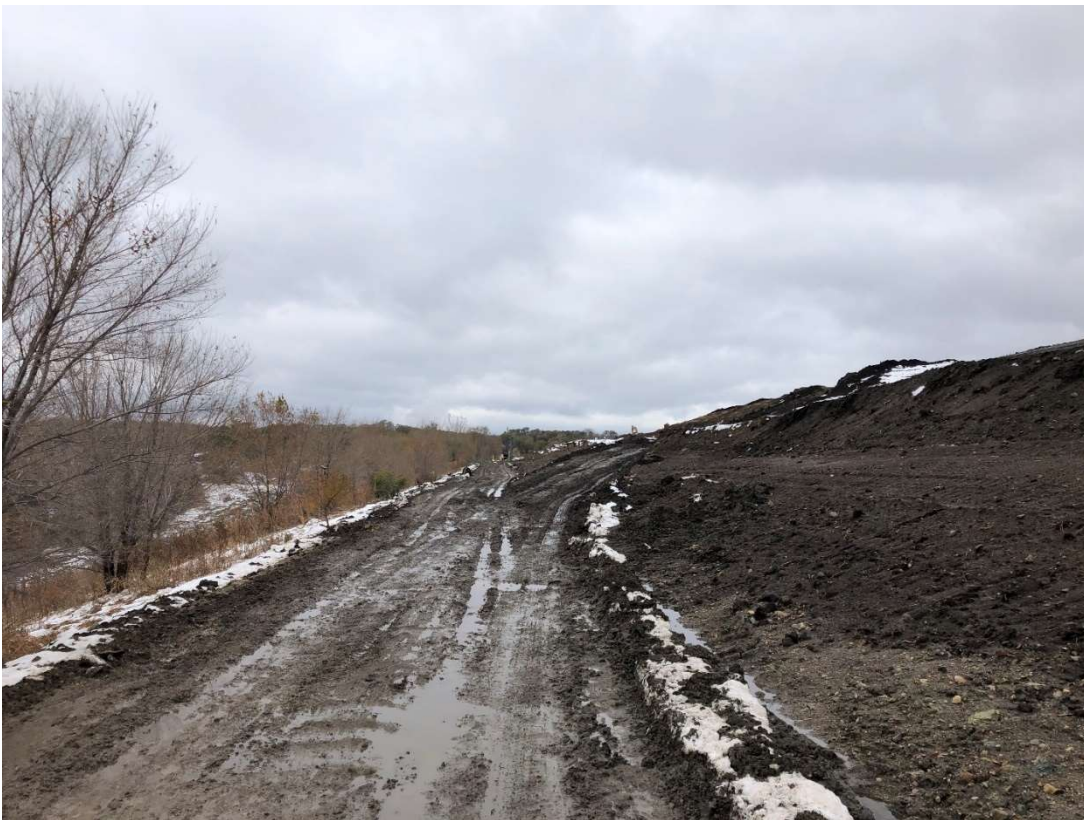
Location 7 – Looking Northwest, Cell 2C Southwestern Slope, Anchor Trench, and Road
