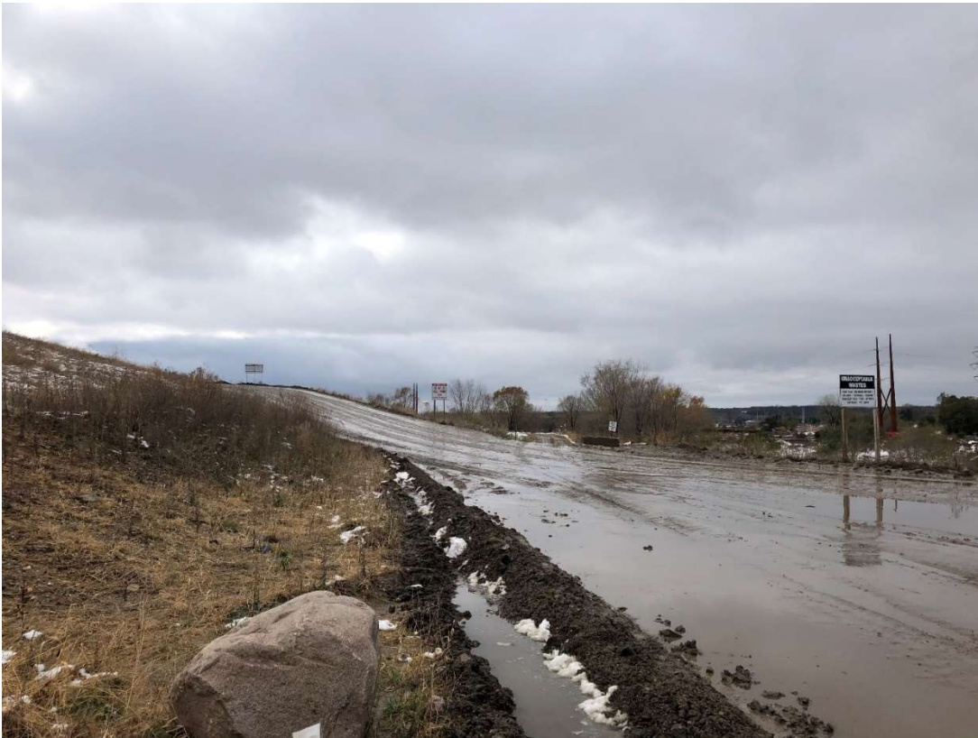
Location 12 – Looking Southwest, Cell 2A Northwest Waste Slope and Anchor Trench
