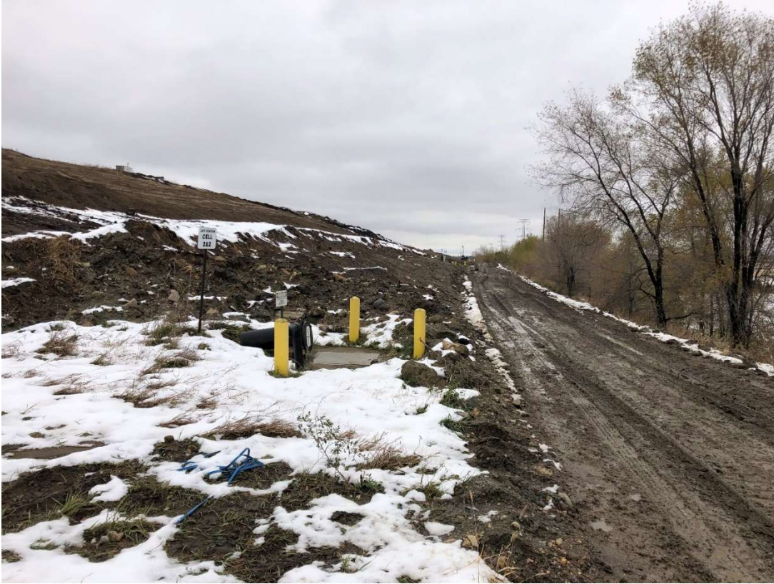
Location 10 – Looking Southeast, Cell 2B Southwestern Waste Slope and Perimeter Road
