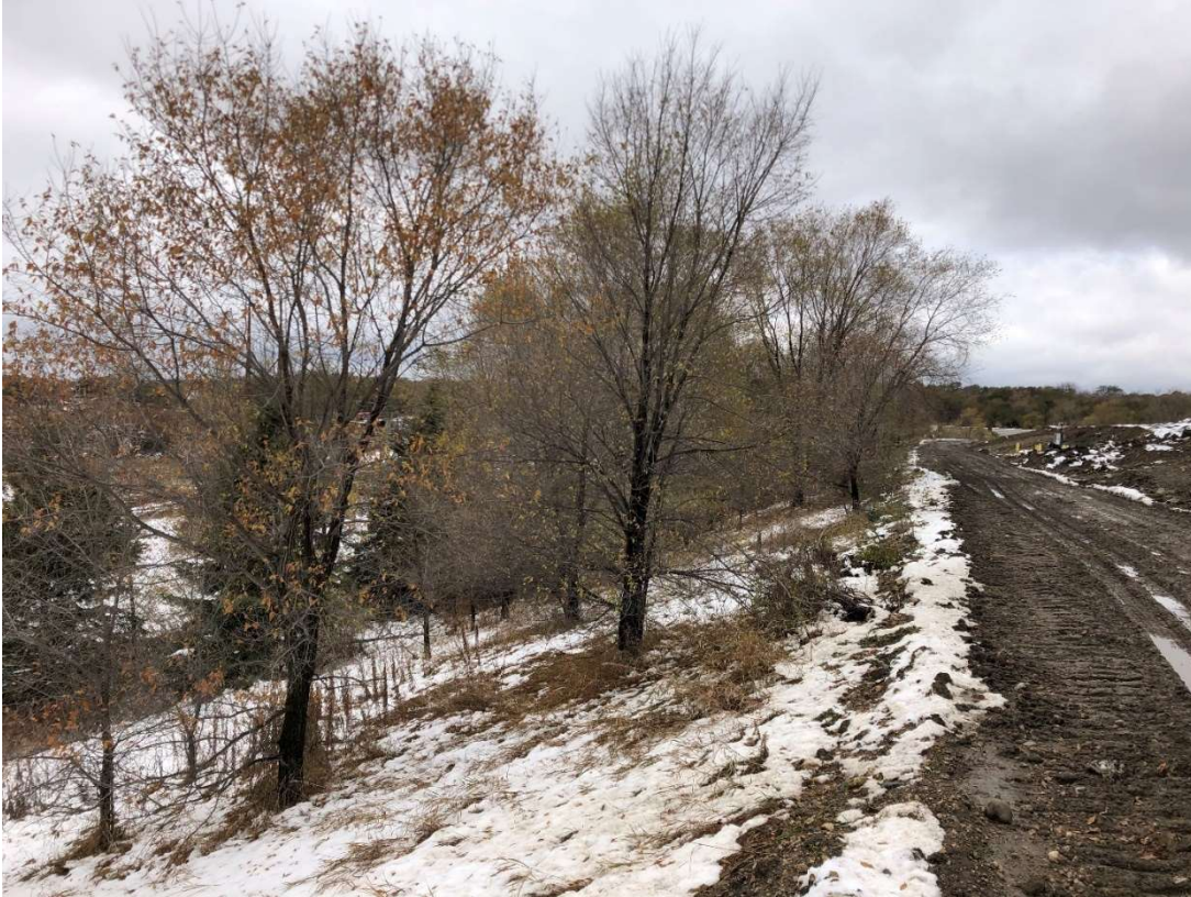
Location 9 – Looking Northwest, Cell 2B Southwestern Berm
