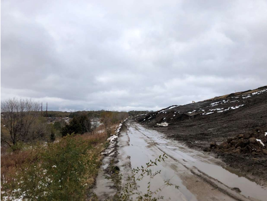
Location 6 – Looking North, Cell 2D Berm
