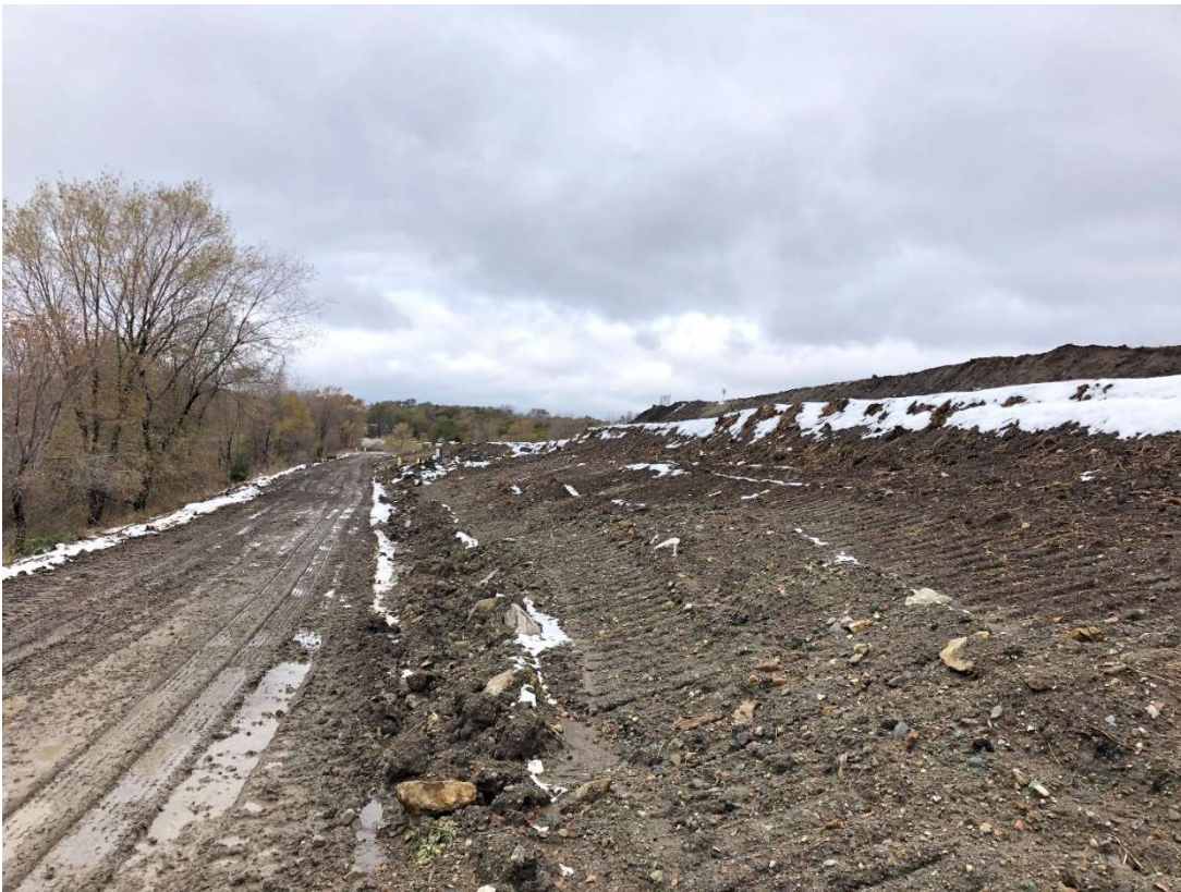
Location 9 – Looking Northwest, Cell 2B Southwestern Waste Slope and Anchor Trench
