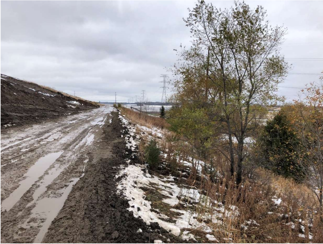
Location 7 – Looking Southeast, Cell 2D Berm
