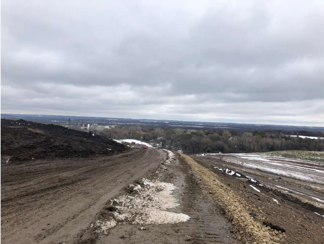
Location 4 – Looking Northeast, Phase 3F Liner Limit
