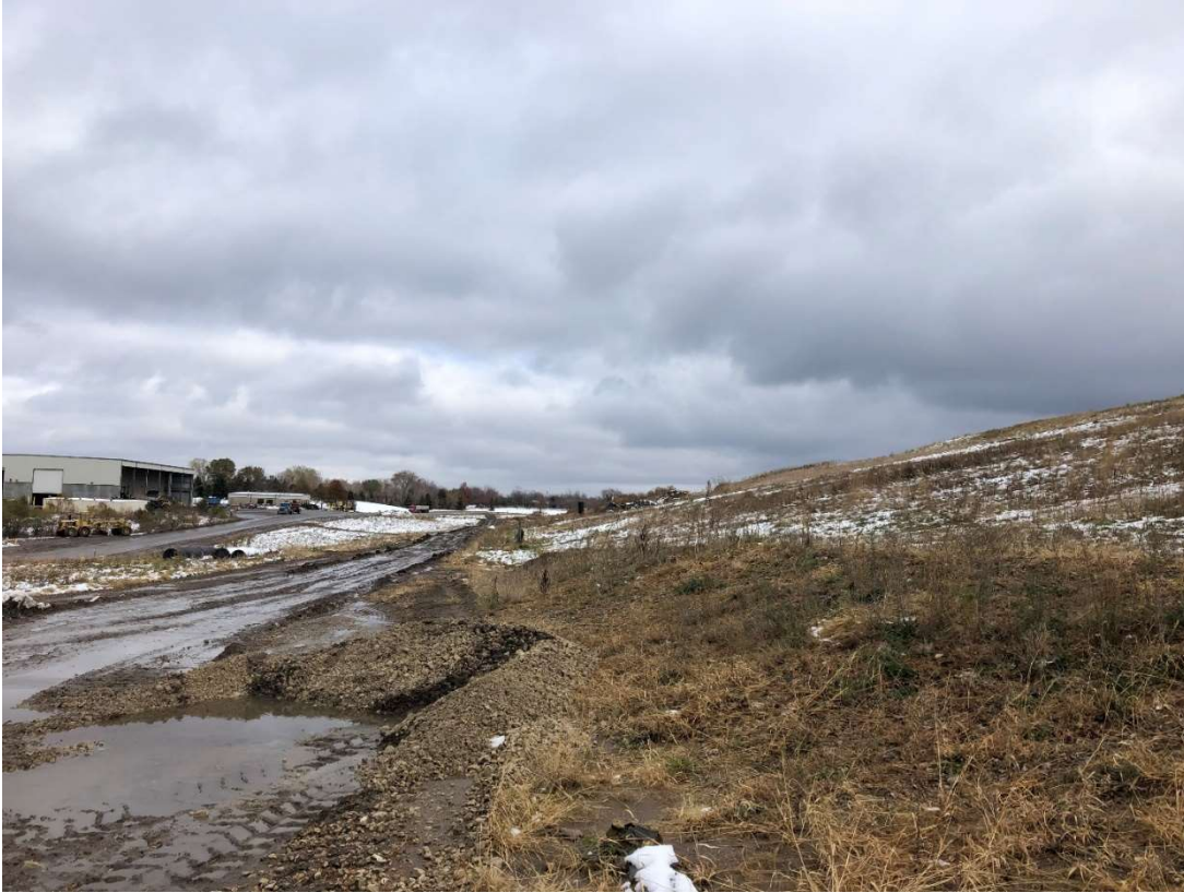
Location 12 – Looking Northeast, Cell 1 Northwestern Waste Slope
