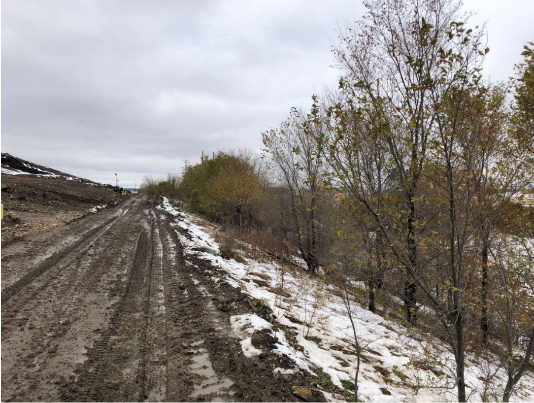
Location 9 – Looking Southeast, Cell 2C Southwestern Berm
