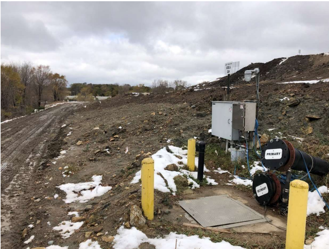
Location 10 – Looking Northwest, Cell 2A Southwestern Waste Slope and Perimeter Road
