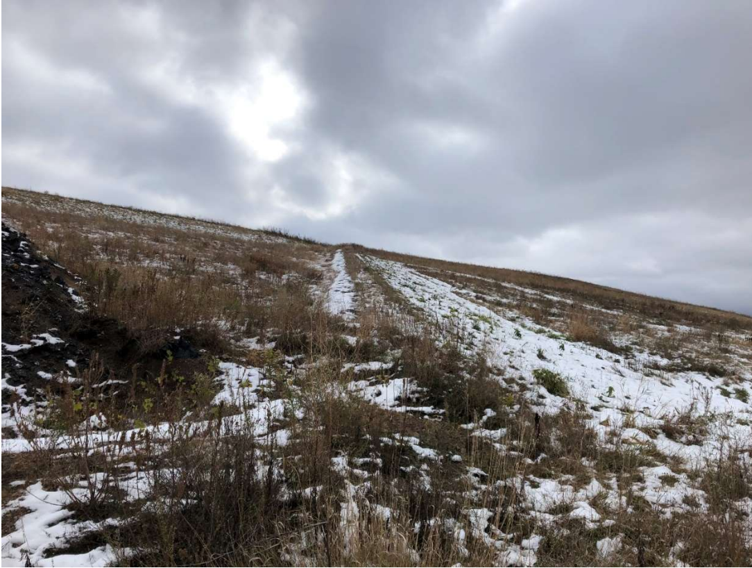
Location 13 – Looking South, Edge of Cap over Cell 1, Limit of Industrial Waste (CCR)
