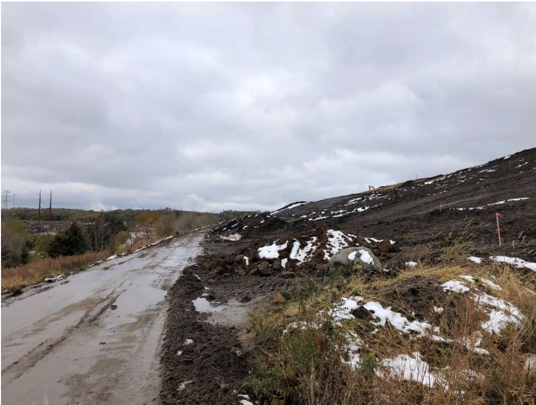
Location 6 – Looking Northwest, Cell 2D Southwestern Slope and Perimeter Road
