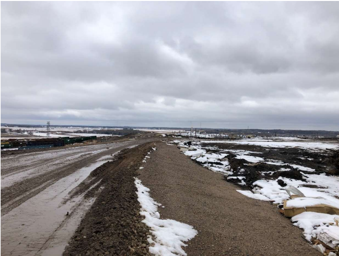
Location 4 – Looking Southwest, Phase 3F Liner Limit
