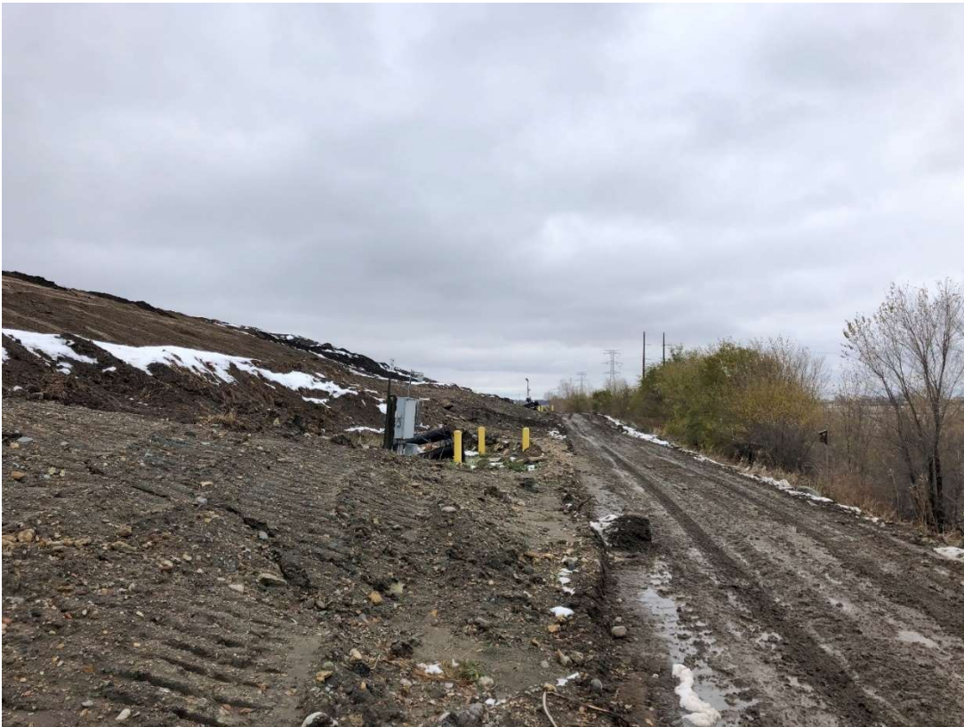
Location 9 – Looking Southeast, Cell 2C Southwestern Waste Slope and Anchor Trench
