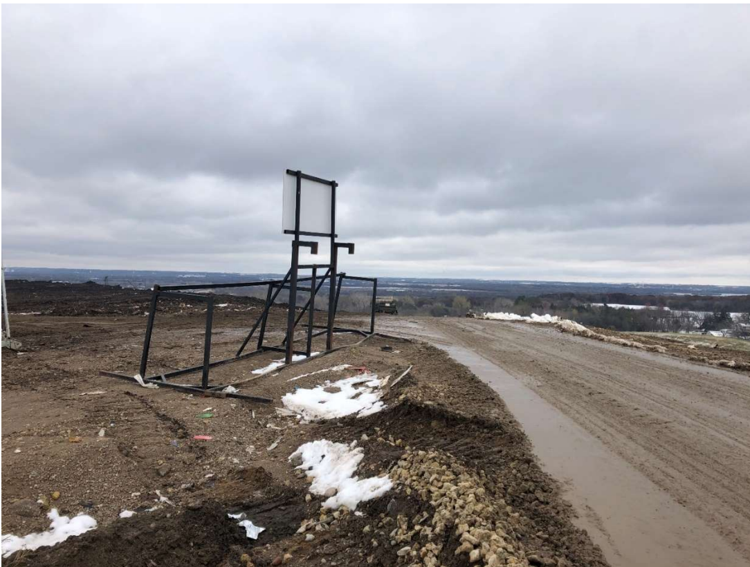
Location 5 – Looking Northeast, Phase 3F Liner Limit
