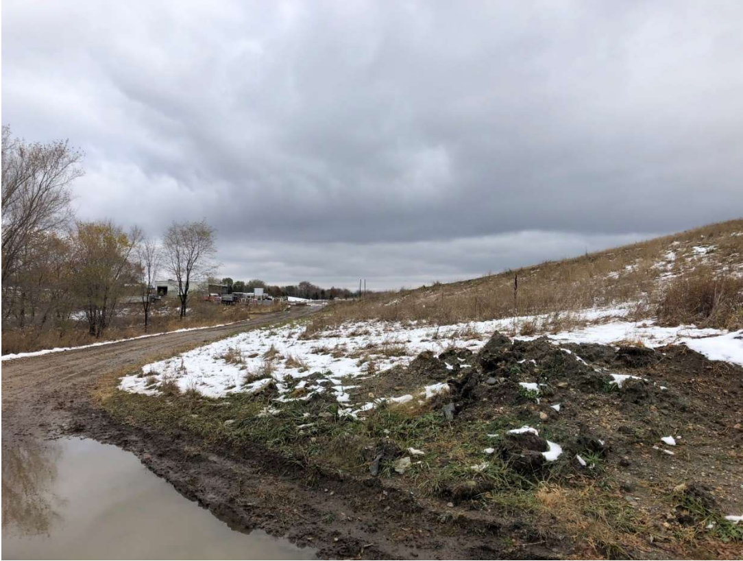
Location 11 – Looking Northeast, Cell 2A Northwestern Perimeter Road and Anchor Trench
