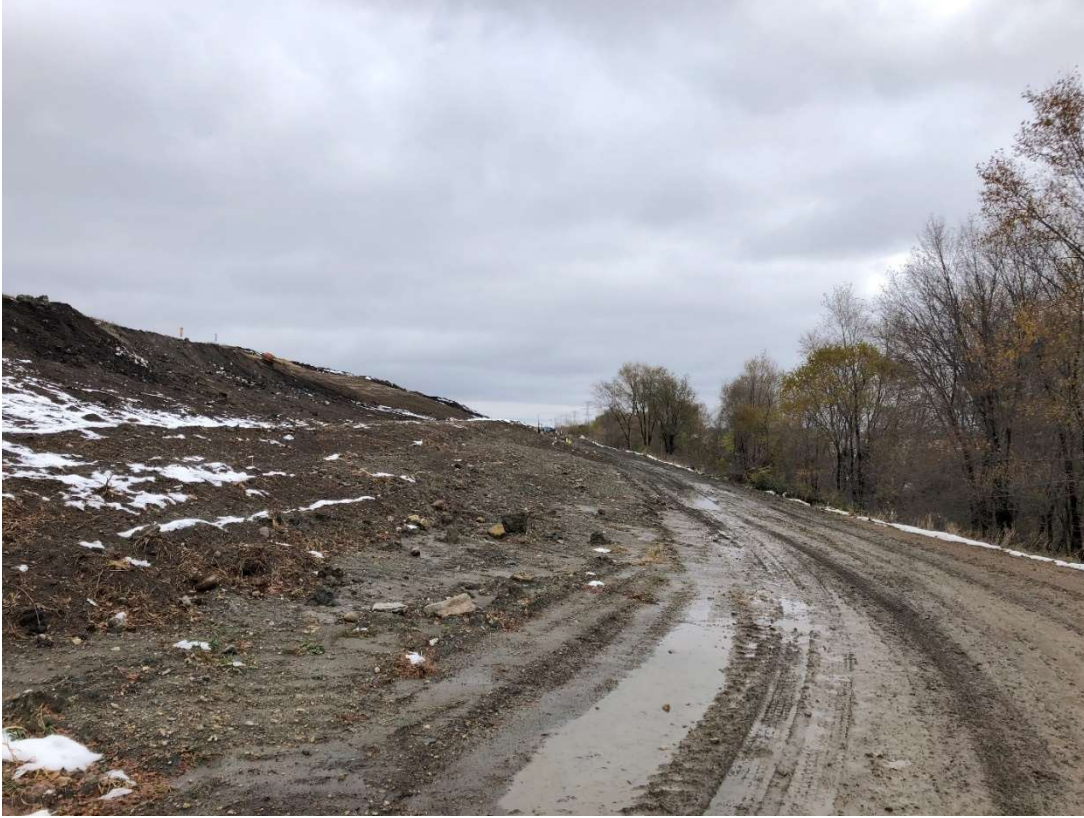
Location 11 – Looking Southeast, Cell 2A Southwestern Waste Slope
