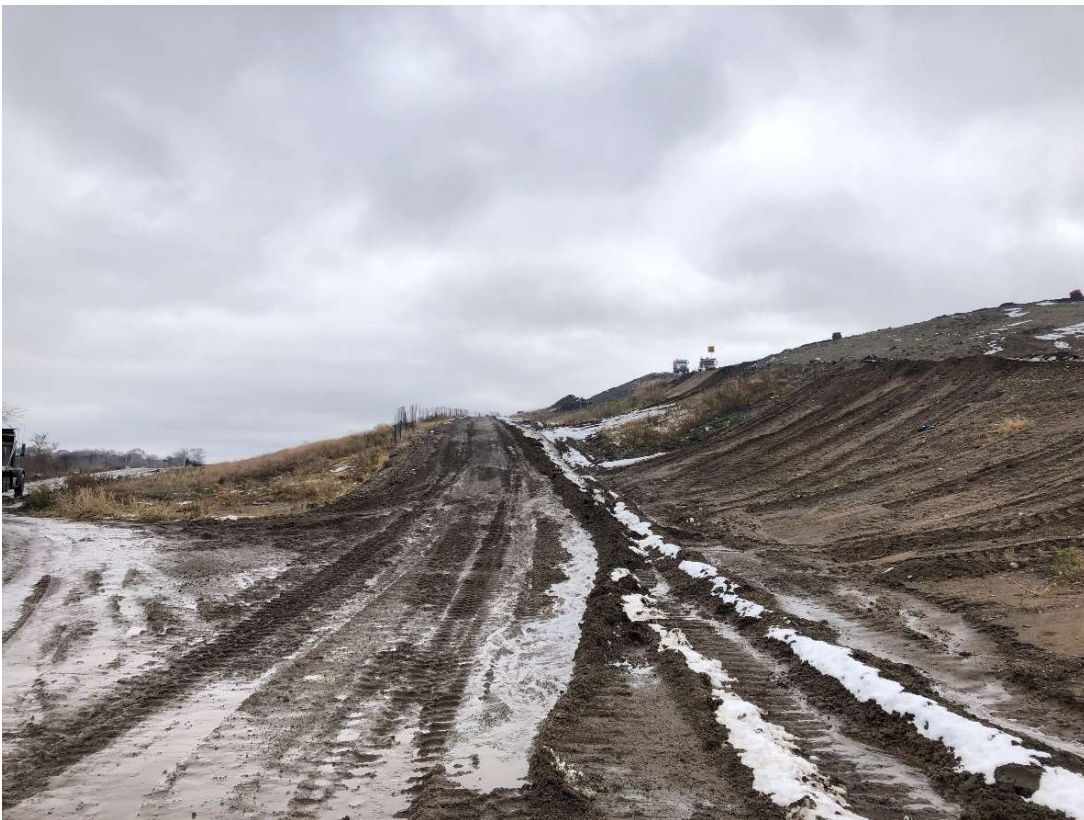
Location 3 – Looking Southwest along Cell 5 Access road/Phase 3F Liner Limit
