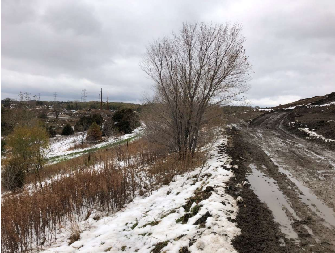
Location 7 – Looking Northwest, Cell 2C Cell 2C Southwestern Berm
