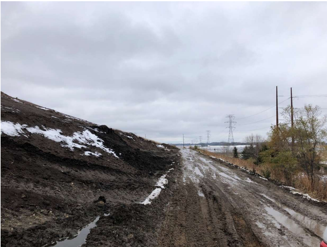
Location 7 – Looking Southeast, Cell 2D Southwestern Slope, Anchor Trench, and Road
