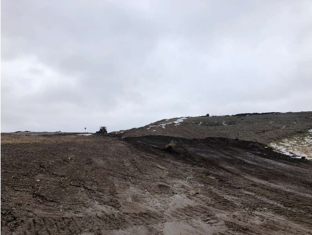
Location 3 – Looking Southwest, Phase 3 East Corner at toe of Interior Access Road
