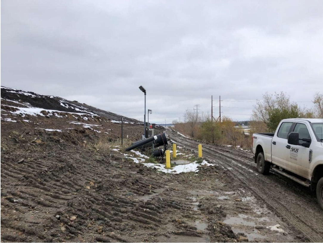
Location 8 – Looking Southwest, Cell 2C Southwestern Waste Slope and Anchor Trench
